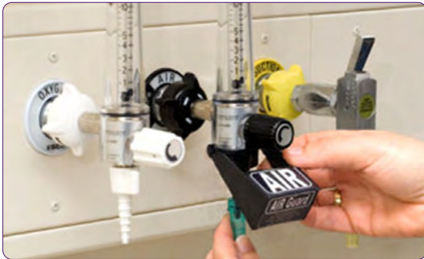
Figure 1 AIR FLOWMETER WITH MOVEABLE FLAP
