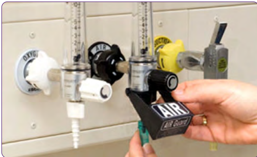
Figure 1 AIR FLOWMETER WITH MOVEABLE FLAP
